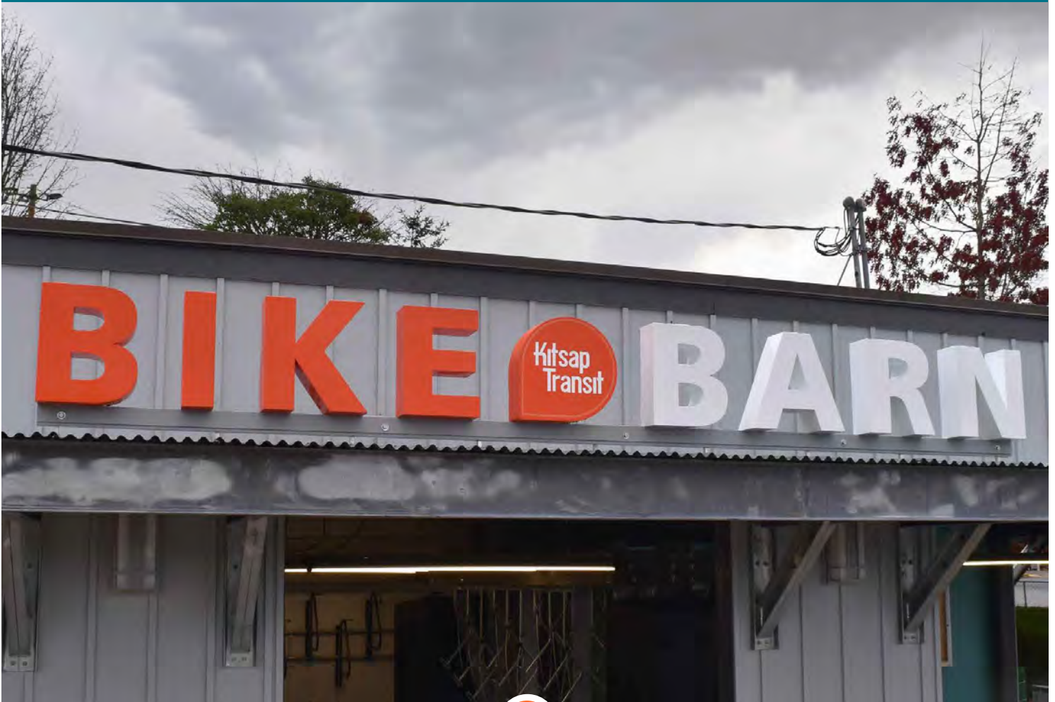
New signage installed during the renovation of the Bainbridge Island Bike Barn.
