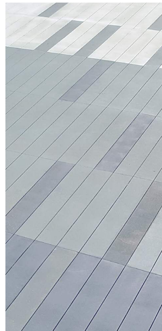
PLAZA SURFACE scored concrete with differentiating tints for plaza + walkways
