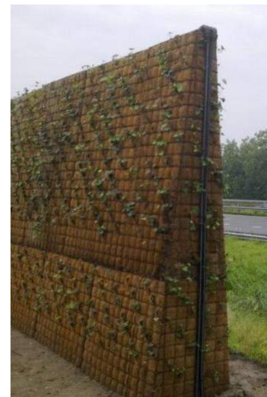
PLANTED / GREEN WALL requires maintenance
