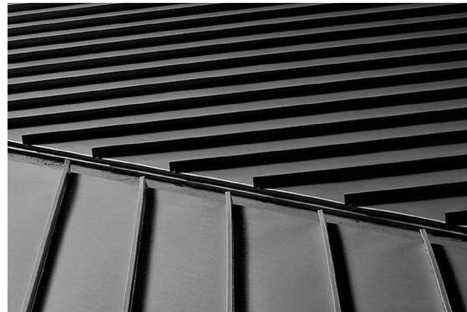
STANDING SEAM METAL canopy roofing
