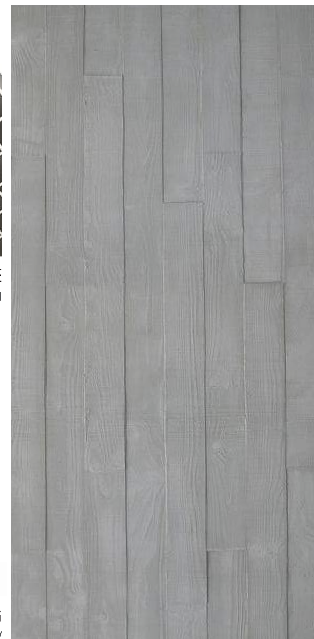
BOARD FORM CONCRETE vertical comfort station volume with graffiti coating
